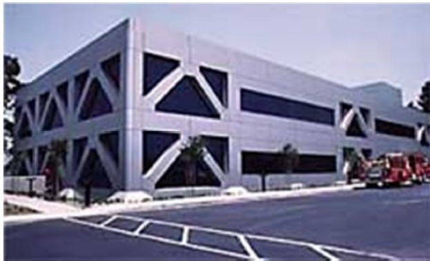
Fire Command and Control Facility, Los Angeles, California
