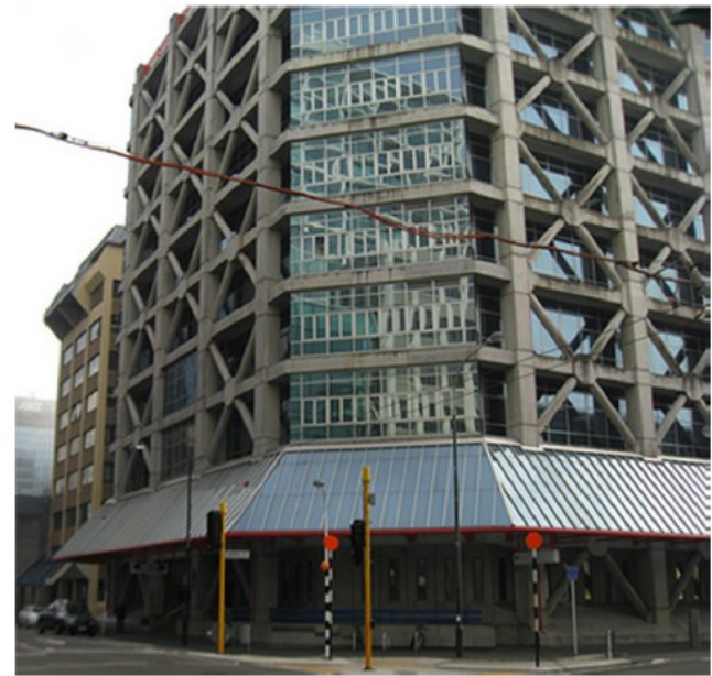
Central Police Station, Wellington, New Zealand
